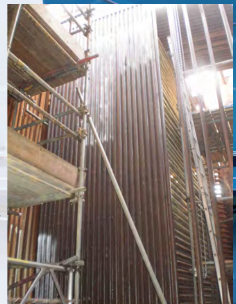
INEOS - Erection of superheater protection wall header
