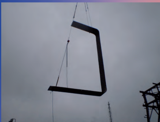
INEOS - Erection of furnace 'D - tube' panels
