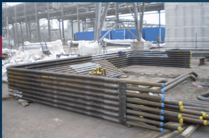
INEOS - Fabricated furnace wall 'D - tube' panels. 17 panels to erect & position inside boiler. Lifted over operational plant & pipe tracks using 160t crane
